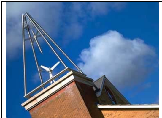
Figure 1: Urban turbine - the spire of St Martha's. Credit: Allan Joyce Architects. A wind turbine was incorporated into the spire of St Martha's Church on the Broxtowe Estate in Nottingham, UK.
